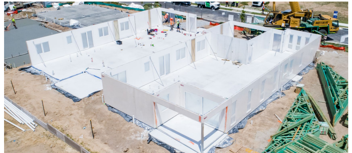
Construction of home with Pro9 walling system
